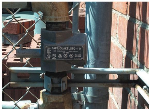
The manufacturer's installation guidelines must be followed to ensure proper SGSV operation. Flow-through SGSVs must be installed in the correct orientation (vertical or horizontal) and gas must flow through the valves in one specific direction. Leveling and rigid bracing to the adjacent structure typically are necessary.
