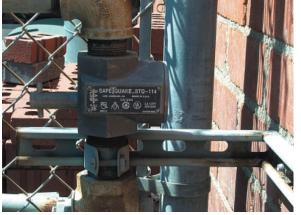
The manufacturer's installation guidelines must be followed to ensure proper SGSV operation. Flow-through SGSVs must be installed in the correct orientation (vertical or horizontal) and gas must flow through the valves in one specific direction. Leveling and rigid bracing to the adjacent structure typically are necessary.
