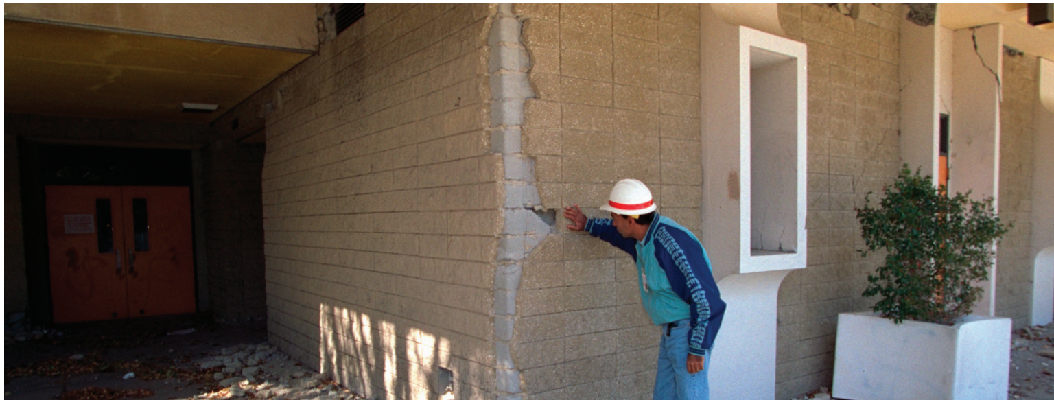
This photo, from the 1994 Northridge, Calif., USA, earthquake, illustrates that, while adequately designed buildings seldom collapse, earthquake damage to structural and architectural systems, and content damage, can result in significant losses. (Photo courtesy of FEMA)
