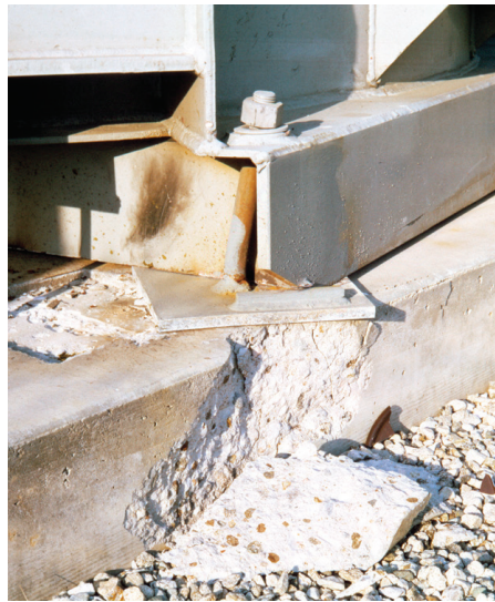
Inadequately designed or installed equipment anchorage may not prevent movement in very severe ground shaking.
