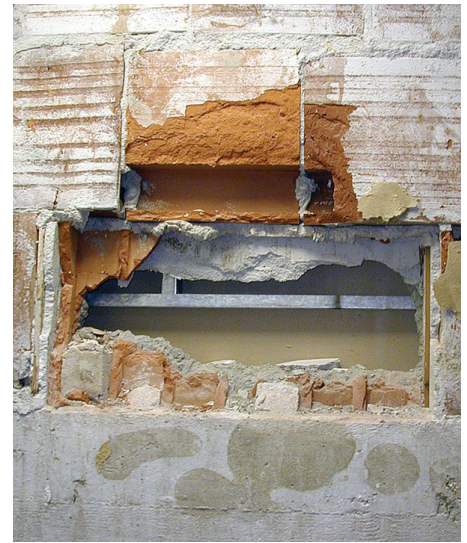
Hollow clay tile partitions (e.g. surrounding stairwells) always perform poorly in earthquakes and should be avoided, even in low seismicity areas.
