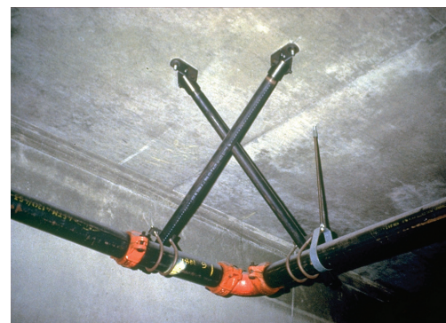
Proper earthquake bracing is essential, for example, where piping changes directions.
